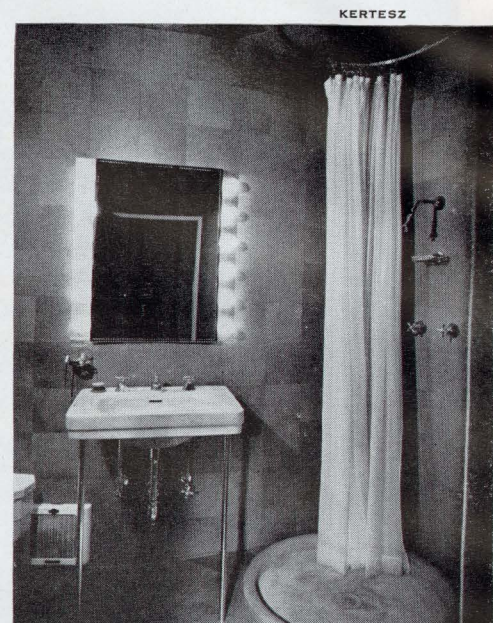
Above: The circular bathroom has cork tile walls, floor and ceiling. The shower, at the right, consists of a recessed concrete base, 34" in diameter, wall fixtures and floor-to-ceiling Koro-seal curtains that operate on a circular track. Left: The living area at night is illuminated by candles, concealed spotlights, the glow of the fireplace and, indirectly, by spotlights set on the roof which light the surrounding trees.
